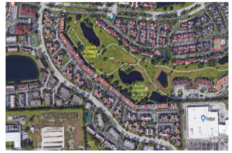
Built in 1981 - 185 units - 2 floors
