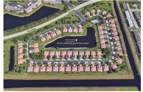
Built in 1994/1997 - 114 units - 1 floor
