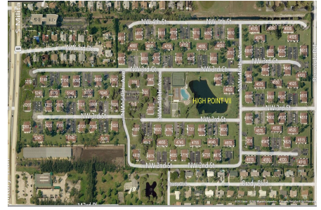
Built in 1977 - 424 units - 1 floor
