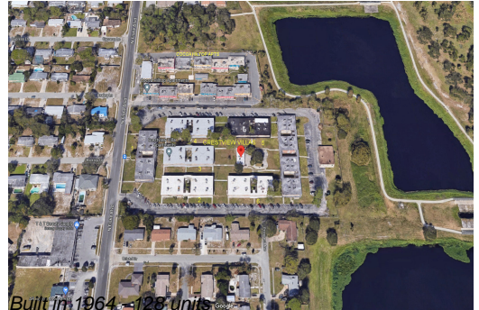
Built in 1964 - 128 units
