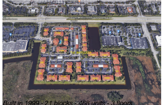
Built in 1999 - 21 blocks ~468 units - 3 floors
