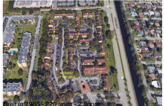
Built in 1986 - 220 units - 302 sq. ft. per unit
