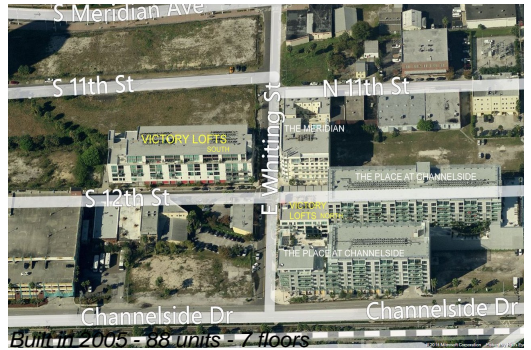
Build in 2005 - 88 units - 7 floors
