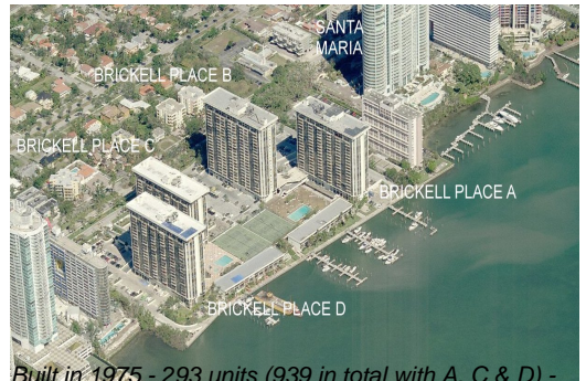
Built in 1975 - 293 units (939 in total with A, C & D) - 26 floors
