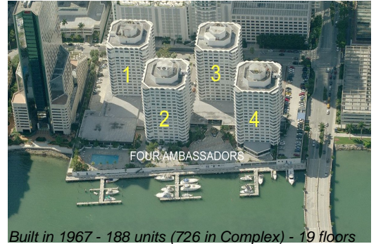
Built in 1967 - 188 units (726 in Complex) - 19 floors
