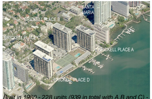
Built in 1980 - 228 units (939 in total with A, B and C) - 23 floors
