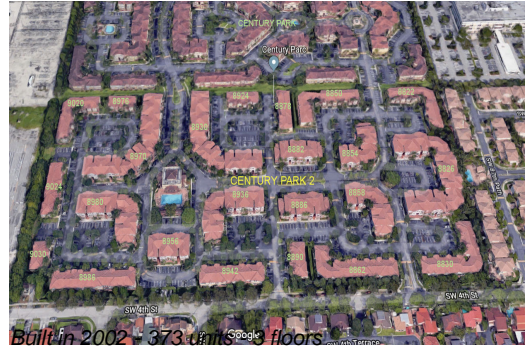
Built in 2002 - 373 units - 300k+ floors
