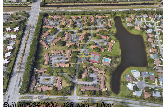
Built in: 1984/1990 - 128 units - 1 floor
