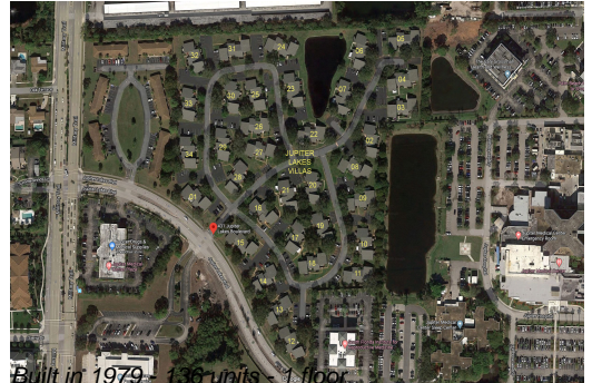
Built in 1979 - 136 units - 1 floor
