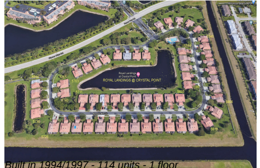
Built in 1994/1997 - 114 units - 1 floor
