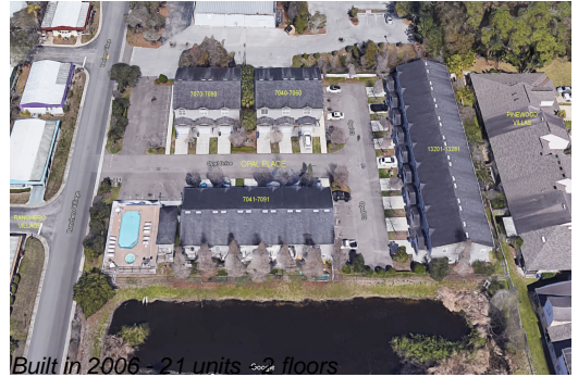
Built in 2006 - 21 units - 2nd floors
